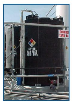
Flexible connections required to preserve warranty; allows for tank expansion / contraction and to reduce pump / piping vibration stress on the tank (page 5)
